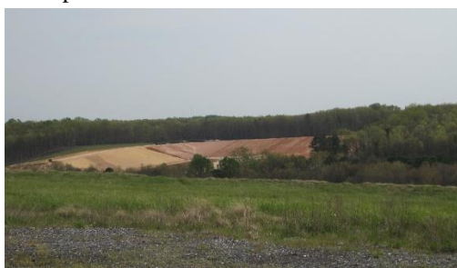
From atop hill – Cell 9 construction
